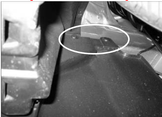
k) From inside the wheel well, remove the retaining clips securing the underbody tray to the chassis.
